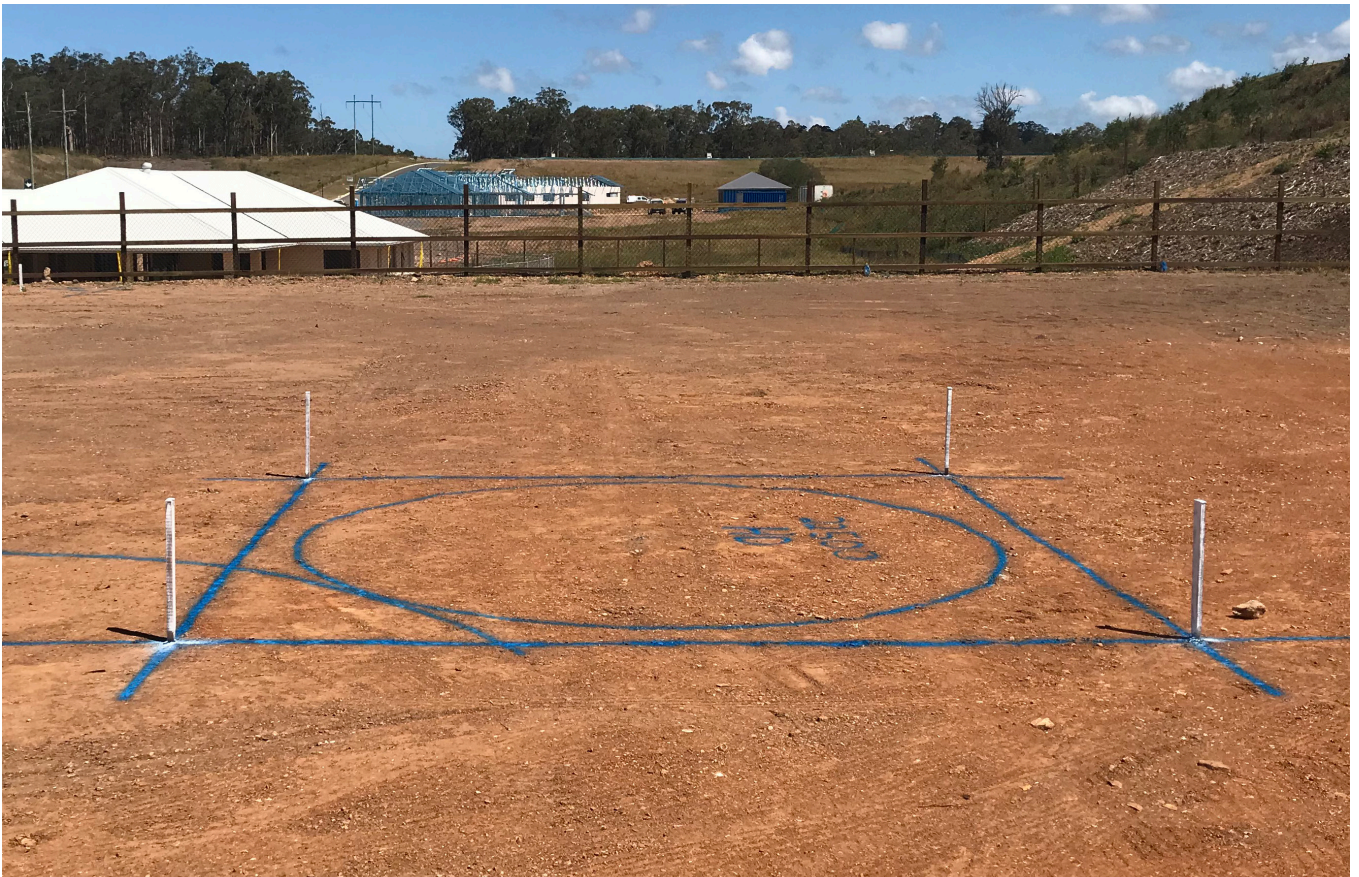
Rainwater Tank Ground Mark out
